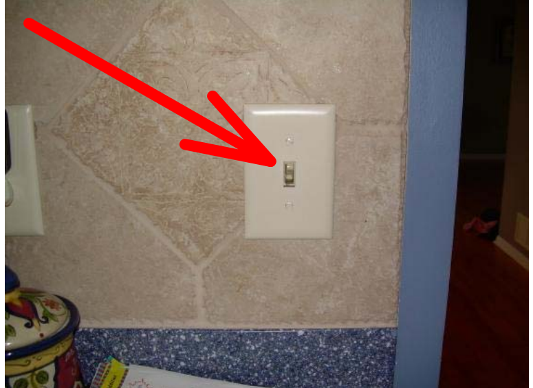
The wall switch to the right of the stove will not operate the can lights when the lights are turned off at the dimmer switch. Recommend evaluation and repairs be made by a qualified electrician.
